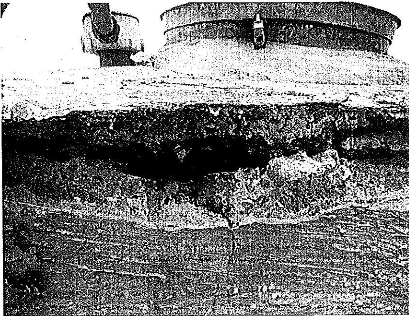
Photo 18 – View of spall on wall-to-cap transition at north end of Tank 2.
