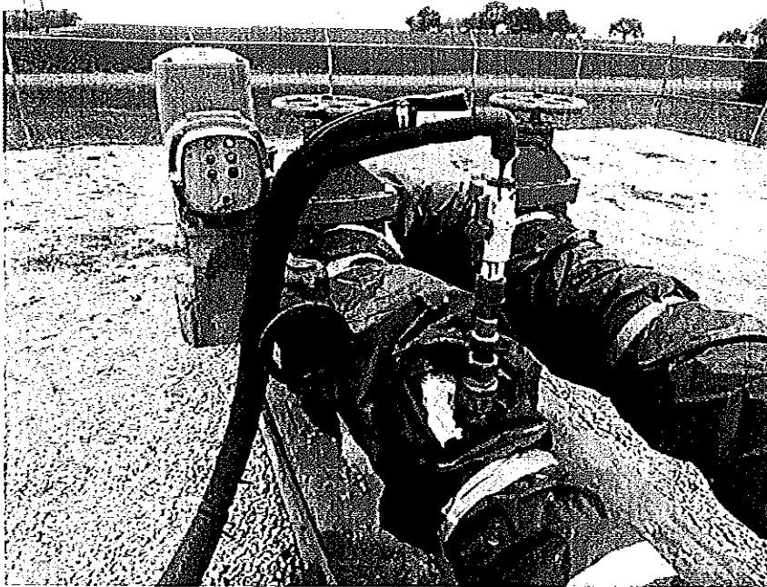
Photo 4 - Close-up view of ancillary components wrapped with insulation, black plastic sheets, and duct tape.
