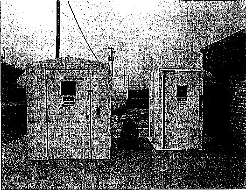
Photo 5 – Ancillary structures containing disinfecting chemicals and equipment.
