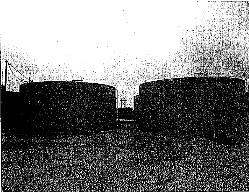
Photo 10 – View of north elevations of Tanks 3 and 4.
